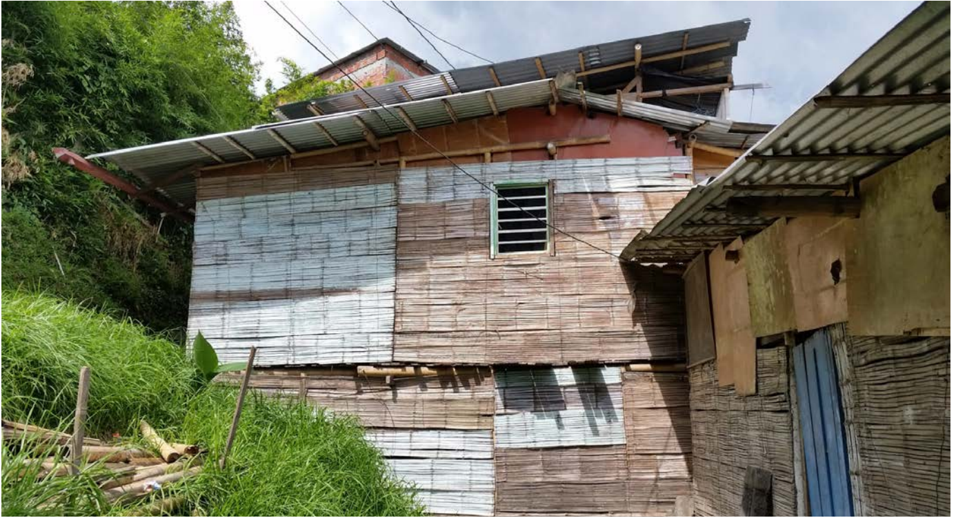
Above: Barrio Los Andres, Manizales, Colombia. Houses in this region have been traditionally constructed from bamboo. The bamboo is often rendered in bahareque (wattle + daub).
