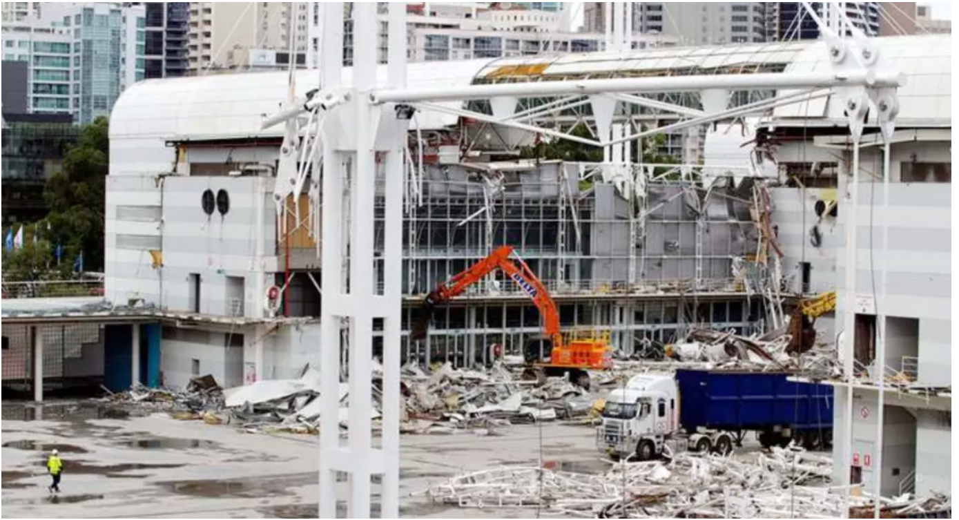
Above: Demolishing the Darling Harbour Exhibition Centre. (Image: Edwina Pickles)
