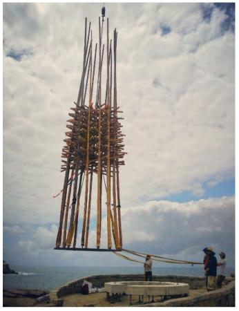
Sitting upon a 4 tonne concrete base, 12m long bamboo poles are attached to it by a steel ring. These poles are joined laterally halfway up the structure with smaller horizontal bamboo members that spiral upwards as a series of triangles.
