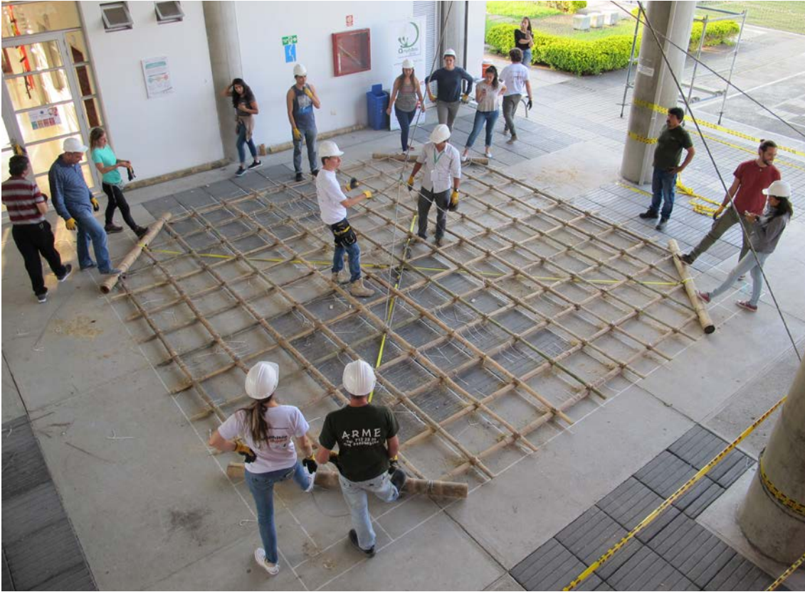
▲ Prefabricating the gridshell on ground Manizales, Colombia Image: Jed Long
