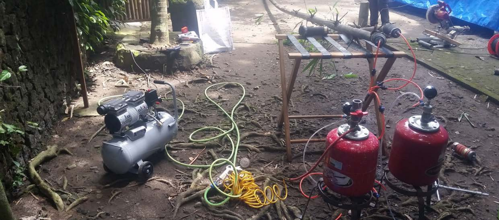
Treating bamboo using the boucherie system ▲ Jogjakarta, Indonesia Image: Jed Long
