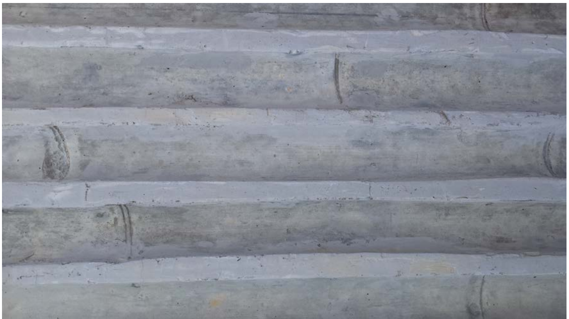
Bamboo Formwork ▲ Ho Chi Minh City, Vietnam Image: Jed Long
