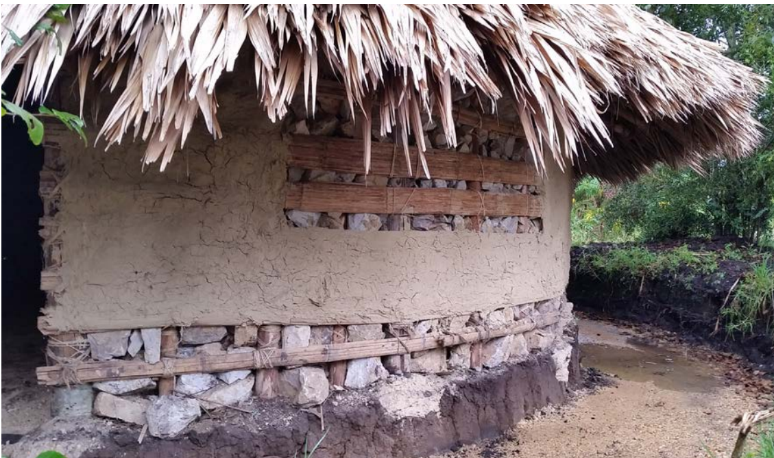
▲ Tradition Maloca wall construction utilising bahareque, bamboo and stone. Tenjo, Colombia Image: Jed Long
