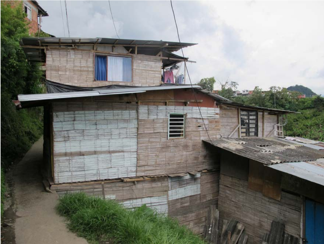
▲ Vernacular bamboo construction traditions continued. The estrias were often painted when a family could not afford to plaster them Manizales, Colombia Image: Jed Long
