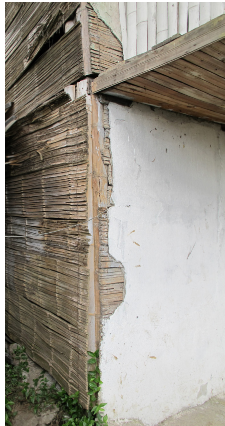
▲ Vernacular bamboo construction traditions continued. The estrias were often painted when a family could not afford to plaster them Manizales, Colombia Image: Jed Long
