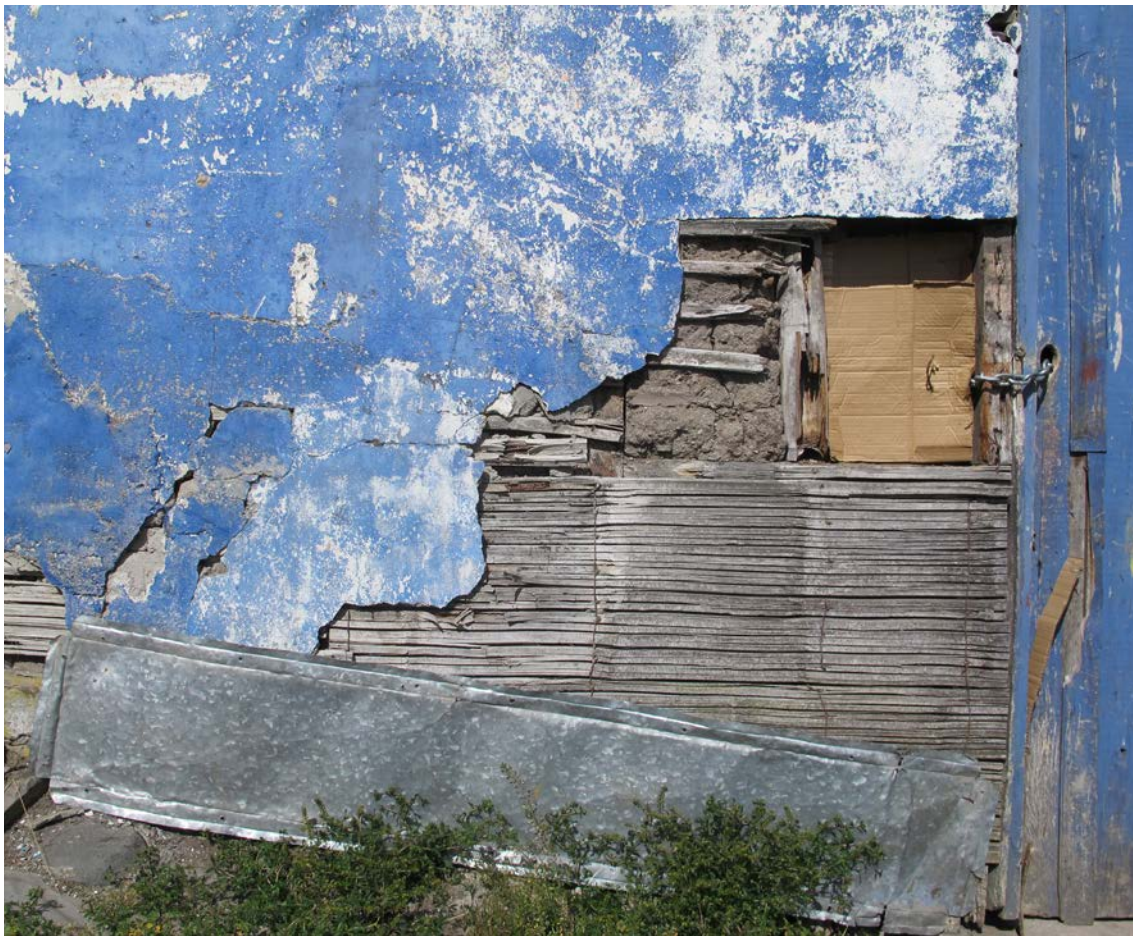
▲ Typical Bahareque Construction Manizales, Colombia Image: Jed Long
