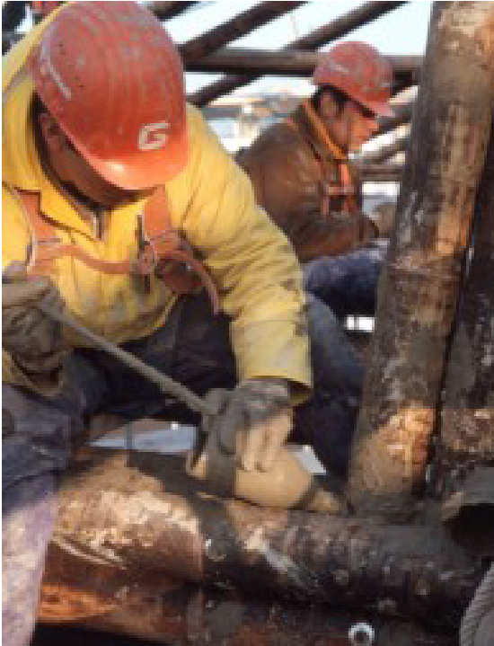
Bamboo Connections, ZERI Pavillion Manizales, Colombia
