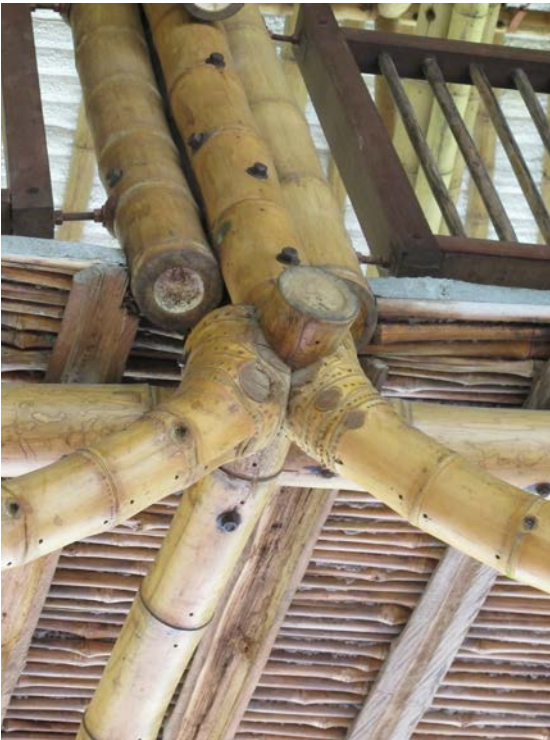
Bamboo Connections, ZERI Pavillion Manizales, Colombia
